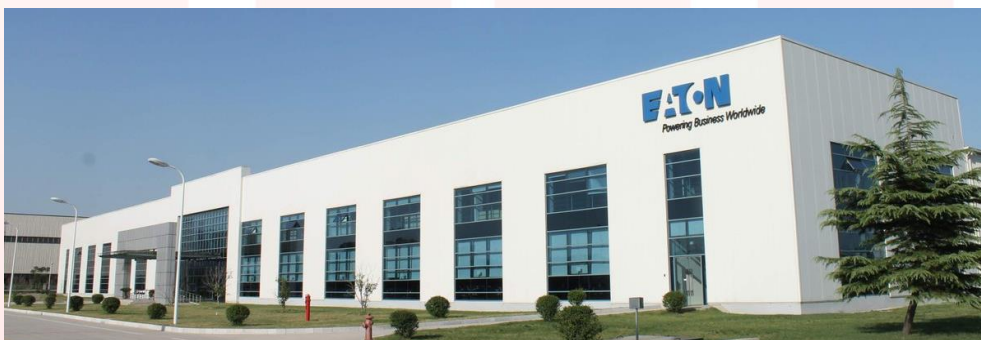
Eaton facilities in Santo Domingo, Dominican Republic.
