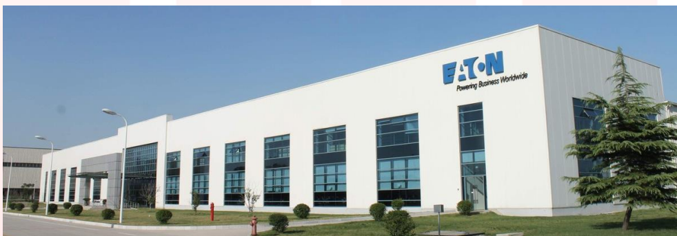
Eaton facilities in Santo Domingo, Dominican Republic.
